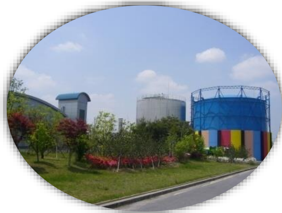
Food Leachate-to-Biogas Plant
