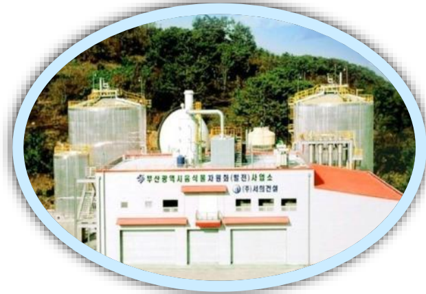
Food Waste-to-Biogas Plant, Busan
