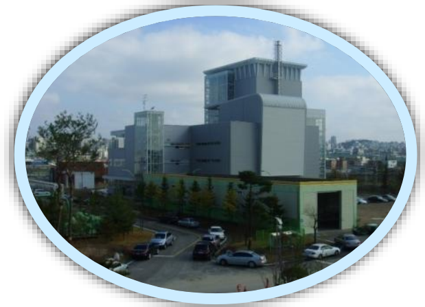
Sewage Sludge-to-Fuel Plant
